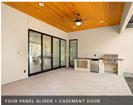
FOUR PANEL SLIDER + CASEMENT DOOR
